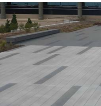
DECORATIVE INTEGRAL COLORED CONCRETE AT ACCESS WALKS AND BREEZEWAYS- SOLID COLOR OR SEA SHELL TOP SEED
